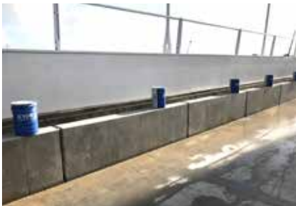
Fig 4 -- Buckets of Xypex Concentrate are pre-positioned along the concrete rail bed that lines the new Bert Swart Bridge in Zuidhorn, Netherlands.
