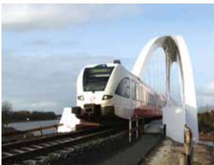
Fig 8 -- The completed Bert Swart Bridge across the Van Starckenborgh Canal in Zuidhorn, the Netherlands, handles two passenger trains per hour on weekdays, as well as freight traffic as needed. The 200-meter long 1,700-ton steel bridge blends architectural beauty and strength. The Xypex-coated concrete rail bed will lower maintenance costs and extend the life of the bridge.
