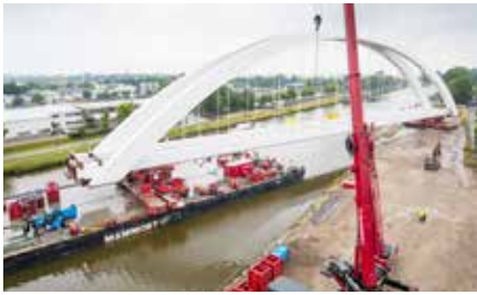
Fig 2 -- As assortment of heavy lift technology is employed by the Mammoet company in order to move one end of the 1,700-ton steel bridge across the canal and into its final position.
