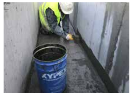
Fig 6 -- A Totech technician applies Xypex Concentrate with a stiff bristle brush along a walkway incorporated into the new Zuidhorn railway bridge.
