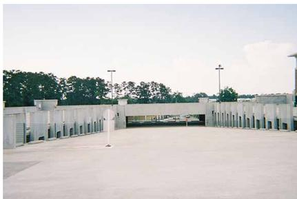
Xypex Admix C-1000 has been used to successfully waterproof the “roof deck” portions of this parking structure in Hammond, Louisiana. The structure consists of precast columns and beams with “double T” panels forming the suspended slabs.
