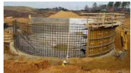
The walls of the thickener tank, used to condense the volume of residual solids, are reinforced, formed and poured.
