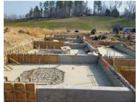
Chemical storage building foundation takes shape. Exterior containment walls are formed and poured using concrete treated with Xypex Admix C-500.
