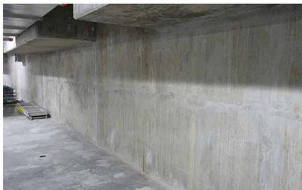
The exterior walls were landed on the slab and the walls had 1" x 1" (25 mm x 25 mm) square profiled preformed control joints space approximately every 20 feet. These construction joints had a PVC waterstop installed to waterproof the expected crack locations. The profile
