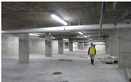
The below grade waterproofing is done using Xypex Waterproofing by Crystallization only. There is no membrane, drainage layer, or drainage assembly used.
