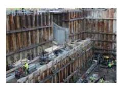
Xypex Admix C-1000 NF was added to the concrete used to create the walls of the two-story deep subterranean Amos Rex art museum. At approximately 14 meters in depth, the concrete walls are subject to continual hydrostatic pressure. Xypex Admix C-1000 NF provides the essential waterproofing protection needed to preserve priceless art in galleries and storage.
