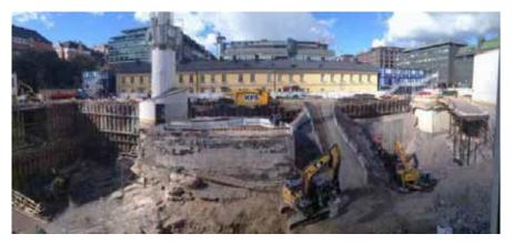
Excavation of Lasipalatsi plaza to accommodate subterranean Amos Rex art galleries and art storage space. Approximately 14,000 m³ of soil and bedrock were removed.
