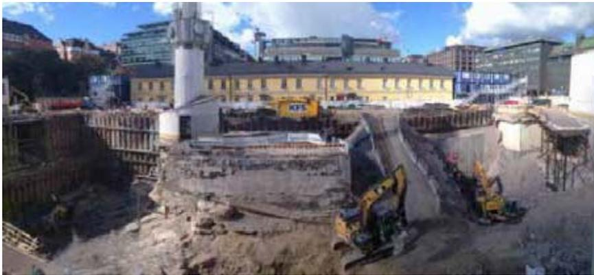
Excavation of Lasipalatsi plaza to accommodate subterranean Amos Rex art galleries and art storage space. Approximately 14,000 m<sup>3</sup> of soil and bedrock were removed.
