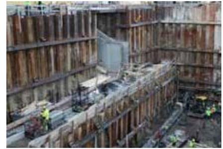
Xypex Admix C-1000 NF was added to the concrete used to create the walls of the two-story deep subterranean Amos Rex art museum. At approximately 14 meters in depth, the concrete walls are subject to continual hydrostatic pressure. Xypex Admix C-1000 NF provides the essential waterproofing protection needed to preserve priceless art in galleries and storage.
