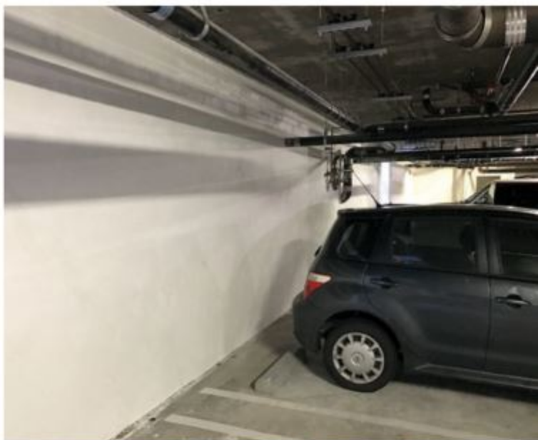
Xypex waterproofing materials successfully sealed this leaking underground parking garage.
