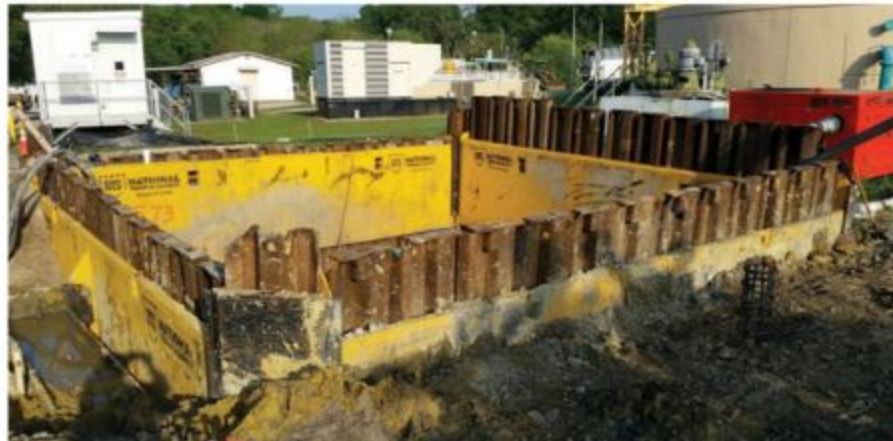
NTS supplies a steel sheeting guide frame system for excavation support.
